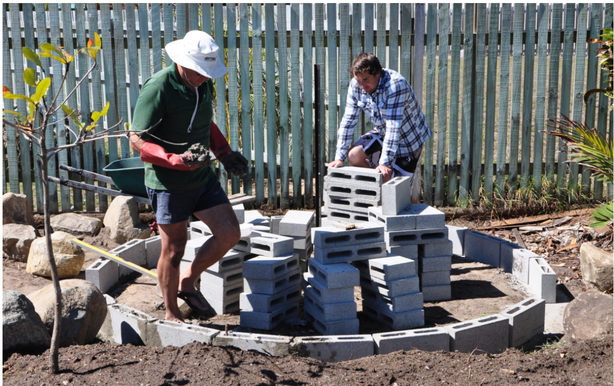
Pic 15 – Block wall base for dome to sit on.
