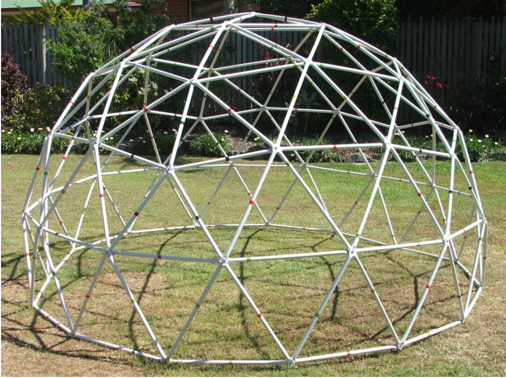
Pic 12 – Structure complete and rigid
