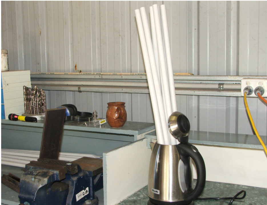
Pic 5 – Softening the conduit ends before flattening in the jig.
